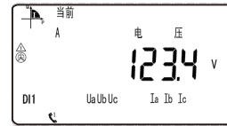
Voltage on A phase is 123.4V
