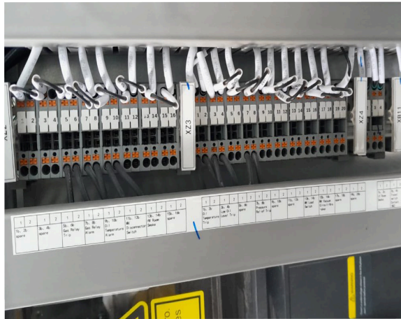
figure 7-2 SCU terminal block
