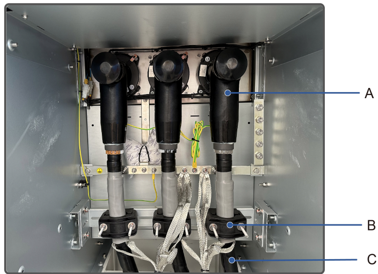
figure 7-4 Cable compartment of the ring main unit
