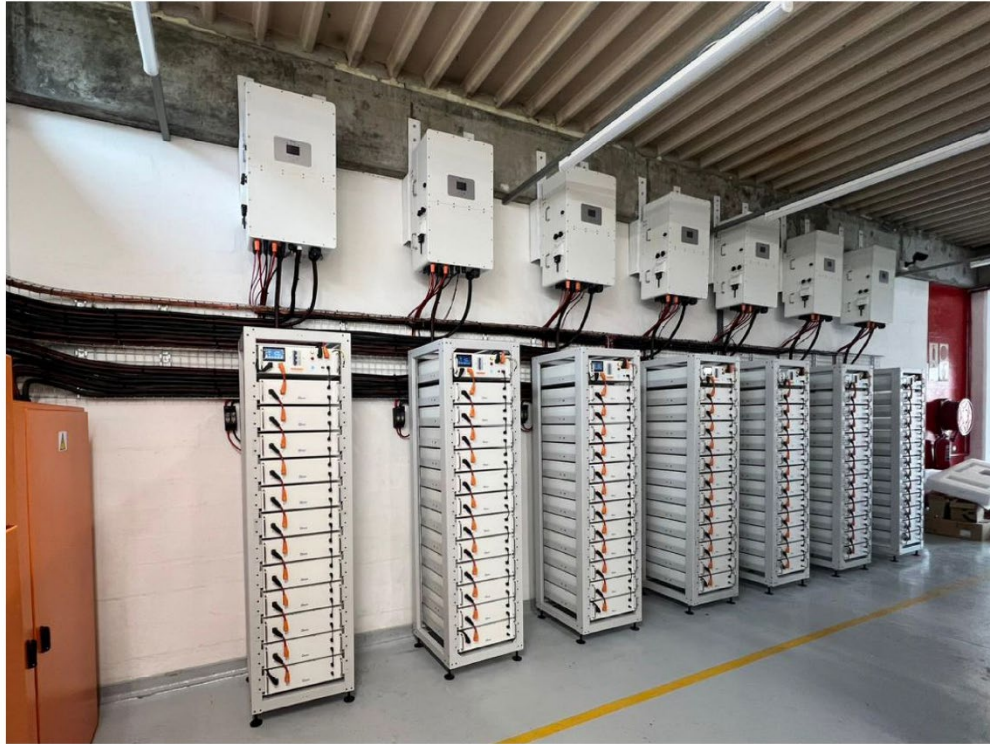
Inverter: SUN-50K-SG01HP3-EU-BM4*7(pcs) Battery: BOS-G
