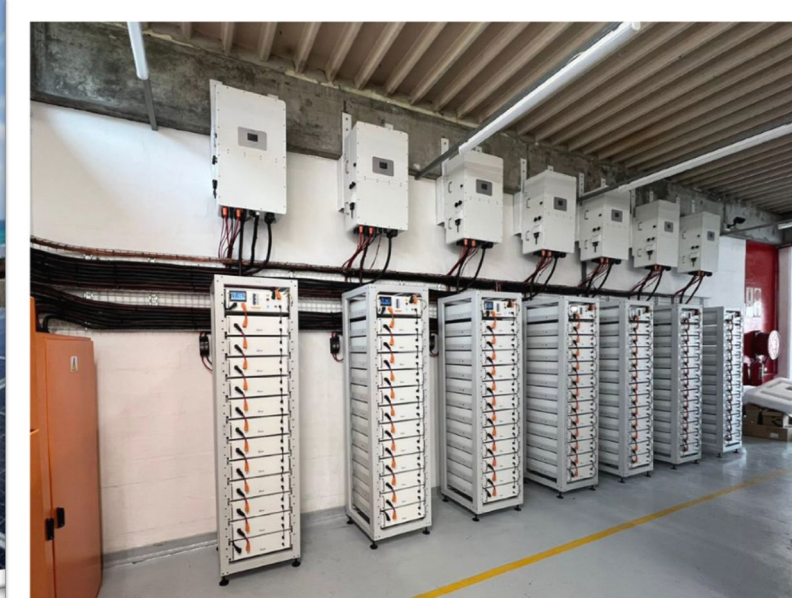
Inverter: SUN-50K-SG01HP3-EU-BM4*7(pcs) Battery: BOS-G
