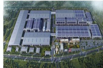
Sichuan Industrial Center EV Cell & Pack 380,000 m 2
