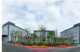
Nanjing Power Industrial Center EV&ESS 1 million m 2
