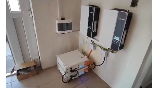
Czech Republic 10kW/10kWh Residential ESS
