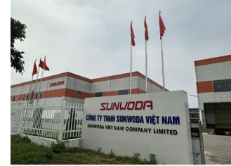
Bac Giang Industrial Center Vietnam 15,100 M 2
